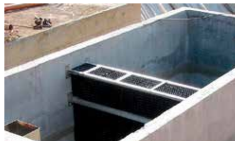
Layout con filtro verticale. Vertical filters installation.
