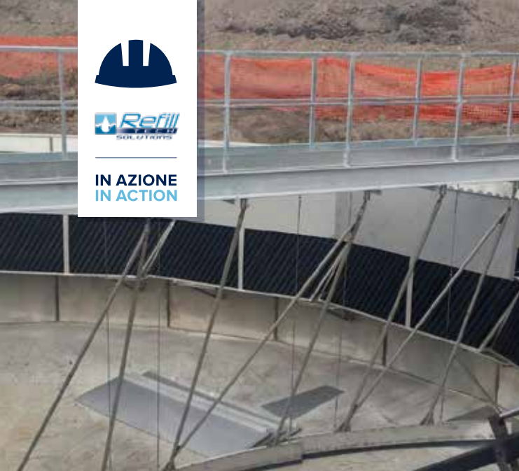
Sedimentatore circolare con LSM50 (PR) Circular clarifier tank with LSM50 (Parma - Italy)
